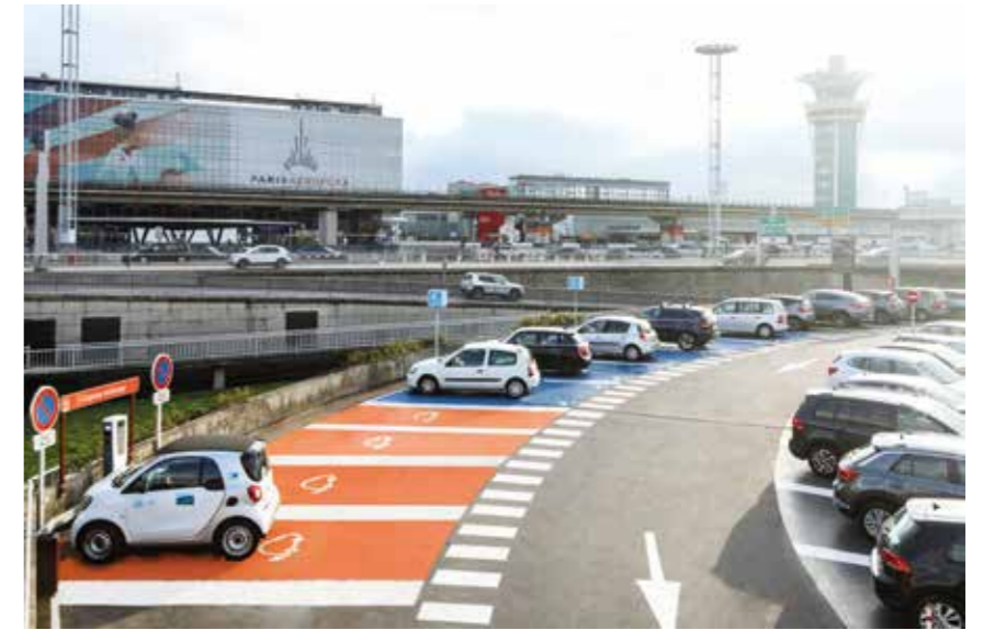
Charging space for electric vehicles at car park P4, Paris-Orly
